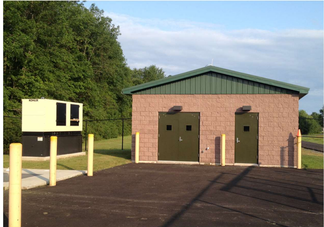
Pump Station – building with emergency generator
